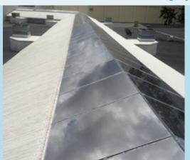
SolarZone SkyLite film transforms overheated mall into a cool comfort zone.
